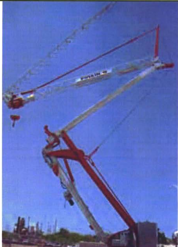
A Coast Crane Company IGO MA21 self erects
