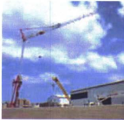
An IGO MA21 from Coast Crane Company builds Coast Crane's new shop
