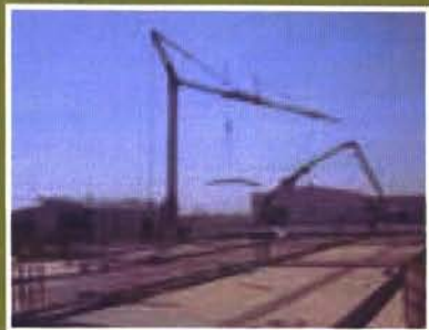
Eagle West supplied Westridge Construction Ltd. a San Marco SMH420 hydraulic self erecting crane to build a $12 million, three storey complex
